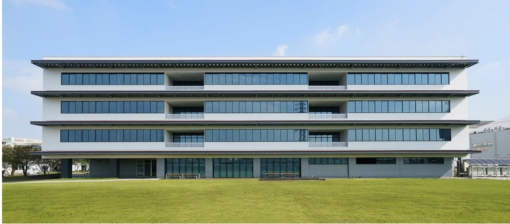
Figure 14: Mitsubishi Electric’s SUSTIE building in Ofuna, Japan.
